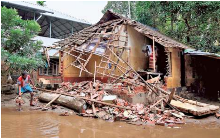
"Rebuilding is different from repairing and demands a paradigm shift in the concept and strategy of development." A scene from Paravur in Kerala after the floods in 2018. ■ REUTERS
